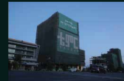
Name - Ayat Lomiyad Site Location - Ayat Building Size - 2B+G+15
